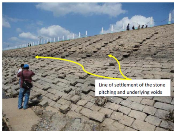
Settlements observed in upstream face of Saddle Dam 1. Source: Technical inspections.
