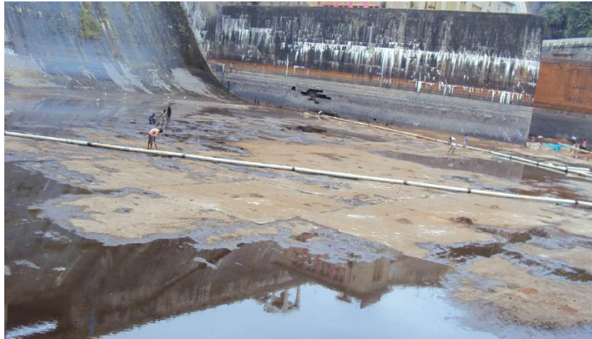
View of the stilling basin after dewatering and cleaning (21 Sept 2017). Source: CSV20170921.
